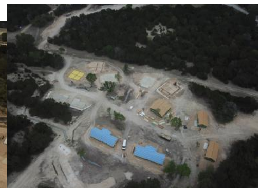
Eagle Trail Project
